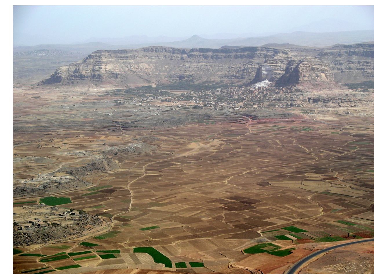
Al-Dhafir – disastrous rock fall in Cretaceous sandstones (Tawilah series)
