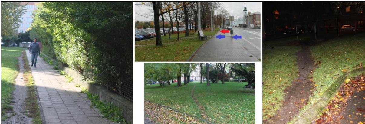
Fig. 3. Left: Maximal pedestrian flow overreaches the capacity of the cobblestone pavement. It caused shortcut in residential district Nové Sady. Middle up: Wrong placement of zebra crossing led to two shortcuts and unused cobblestone pavement in Moravská Ostrava. Middle down: Missing sidewalk around the park force pedestrian walk through the street or shortcut in Poruba part of Ostrava. Right: Playground is not connected with the pedestrian network, thus four shortcuts have been tracked out. (Source: Mudron)
