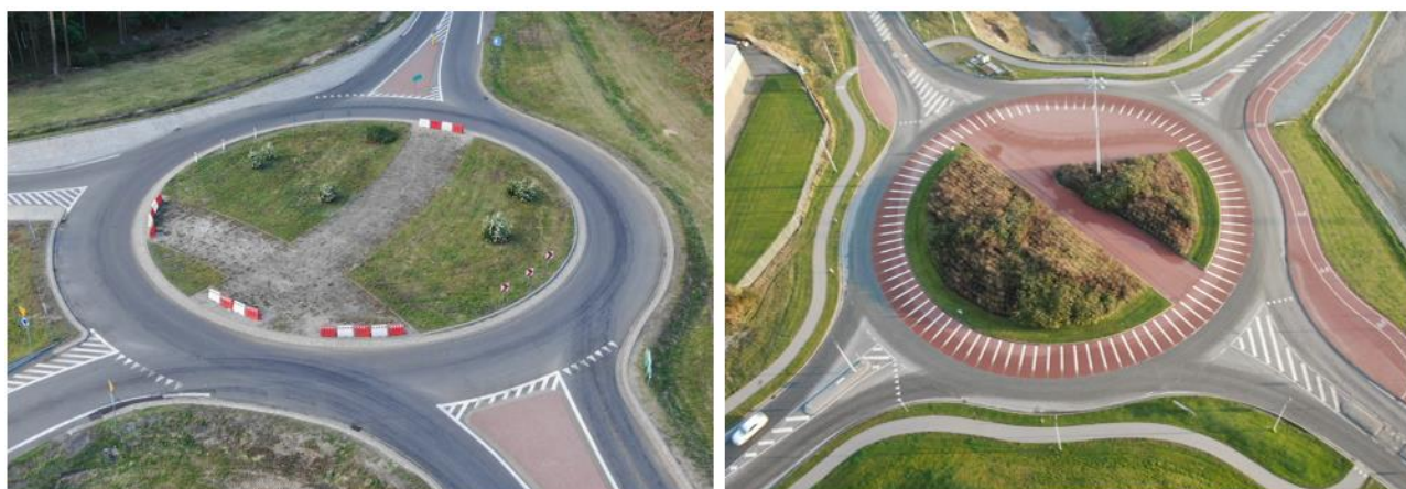
Fig. 4. Modification for passage of the cargo on the roundabout in Poland and roundabout in Denmark
