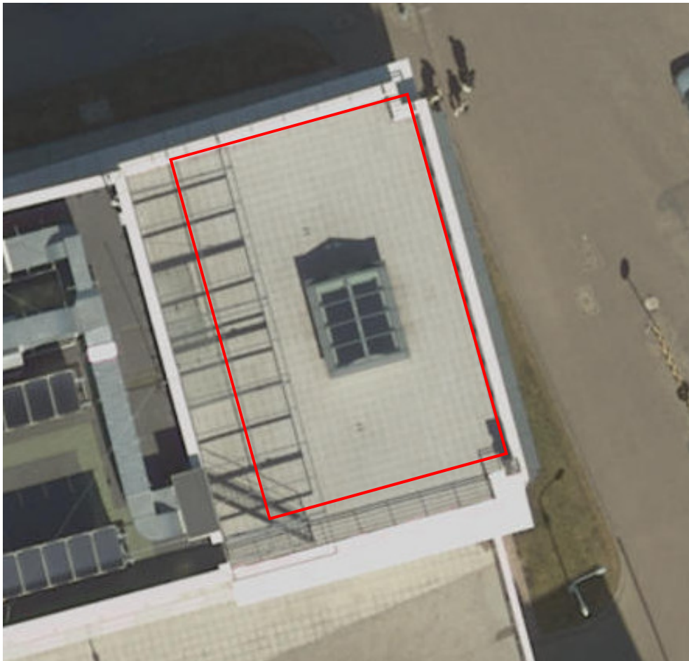
Fig. 2. Test area - terrace of one of the building UPWr (Wrocław, Poland)
